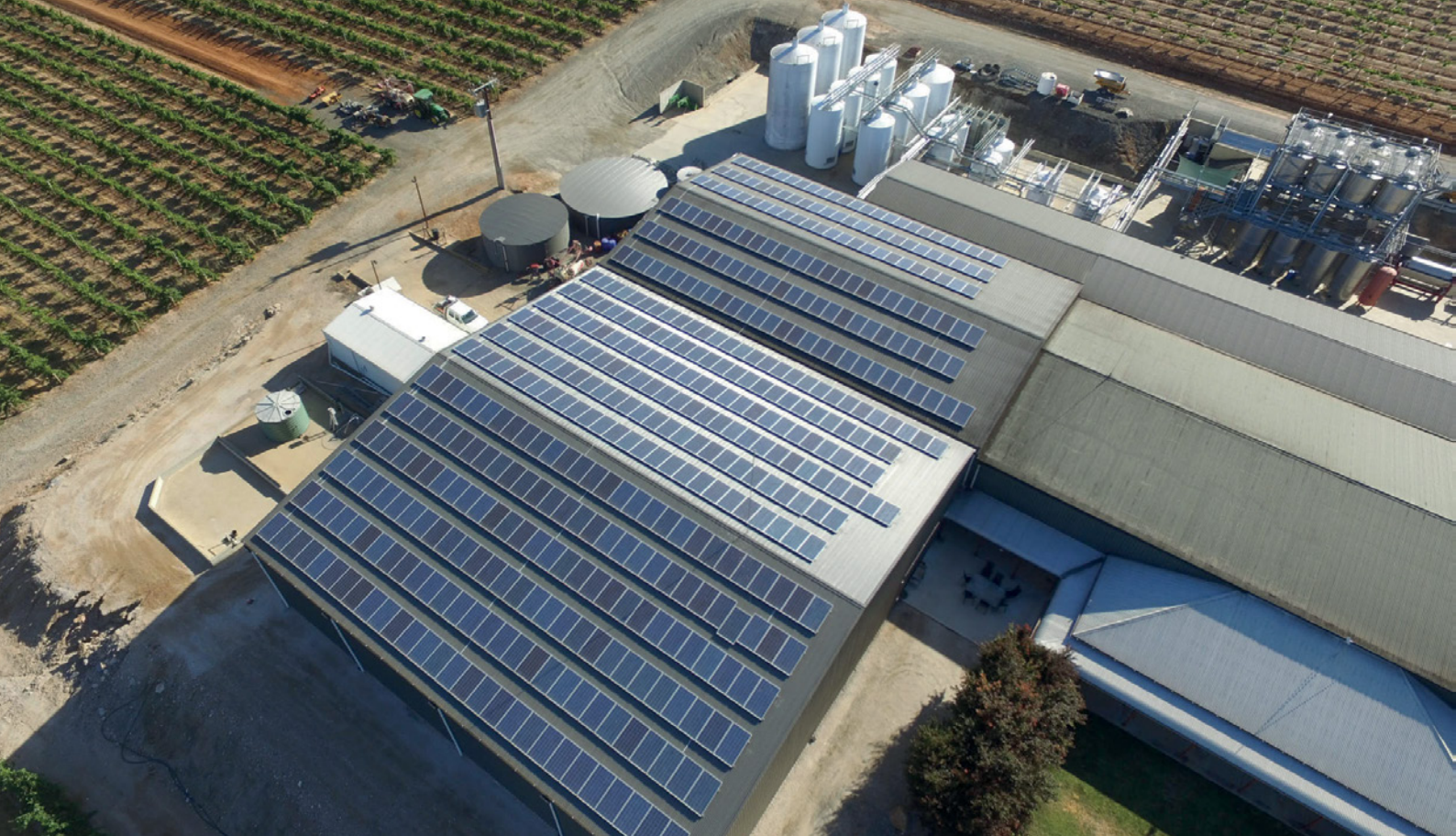
Figure 5: Solar panels on Clare Valley winery in South Australia.
