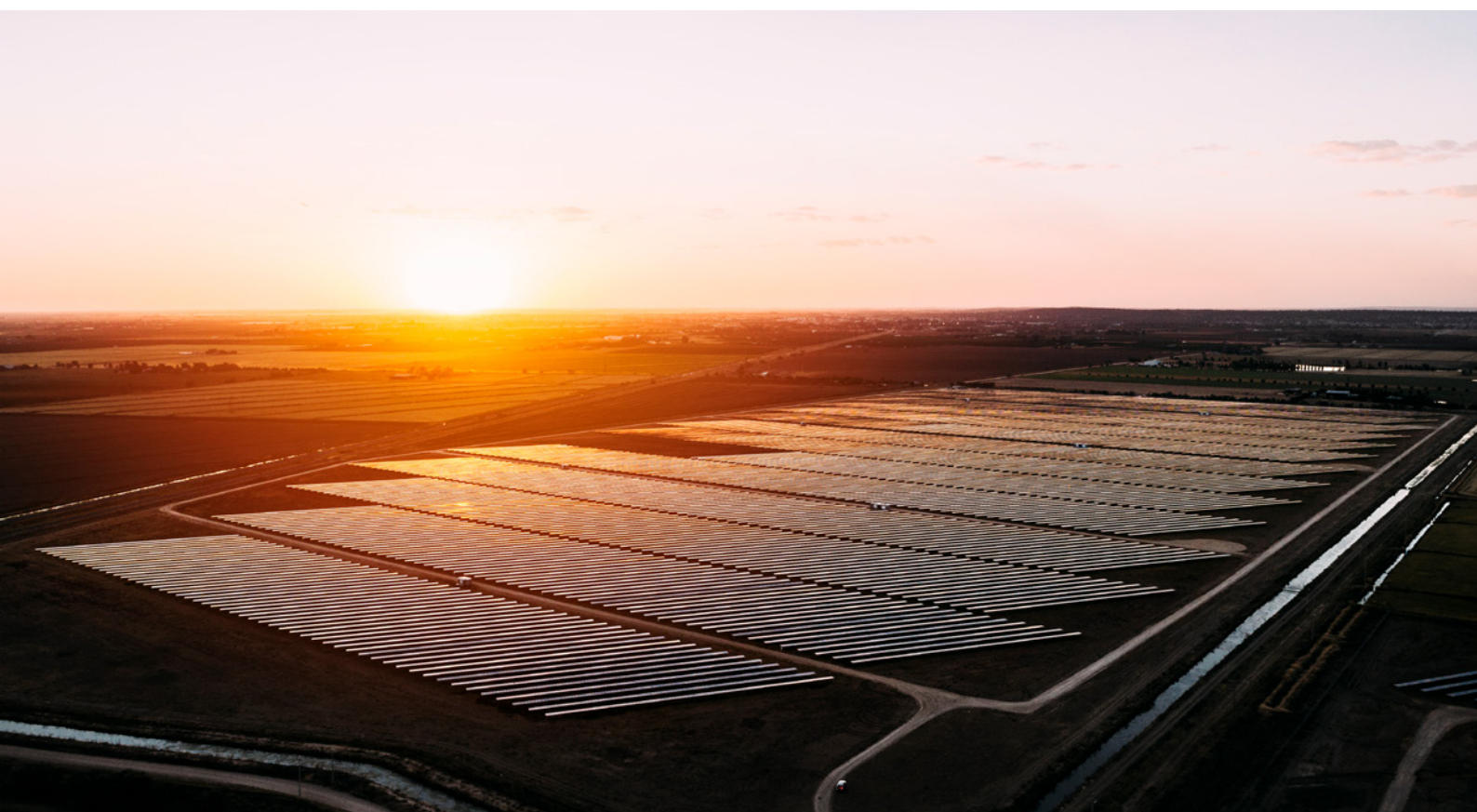
Figure 11: The Griffith Solar Farm is one of a number of large-scale solar farms commissioned in NSW in 2018.
