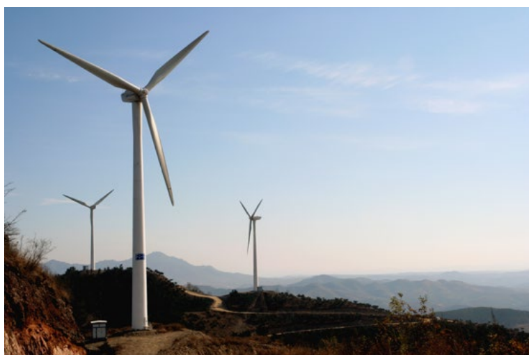
Figure 16: Tangshanpeng Wind Farm in Shandong Province, China.
