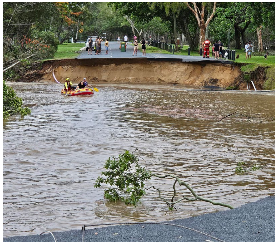
Image 4: Tropical Cyclone Jasper damaged at least 1,863 properties and destroyed 20 of them in Cairns and surrounding areas. The destruction caused an estimated $357 million in insurance losses (Byrne 2024, Insurance Council of Australia 2024).
