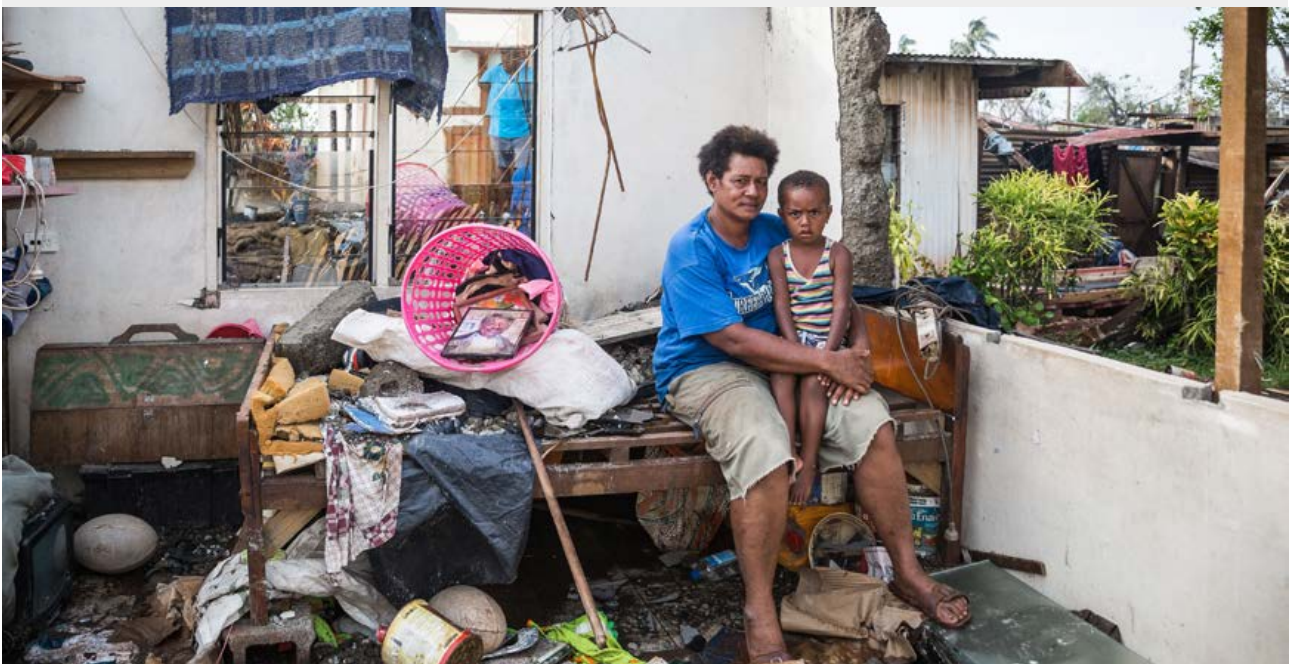
Figure 7: Kalisi holds her son Tuvosa, 3, in the remnants of her house in Ra province, Fiji, after category 5 Tropical Cyclone Winston – the strongest tropical cyclone recorded in the Southern Hemisphere – struck in February 2016. A warming ocean provides more energy for tropical cyclones.
