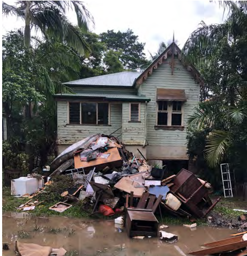
Image 10: Many homes in Lismore, Northern New South Wales were badly damaged in the '2022 Great Deluge'.
